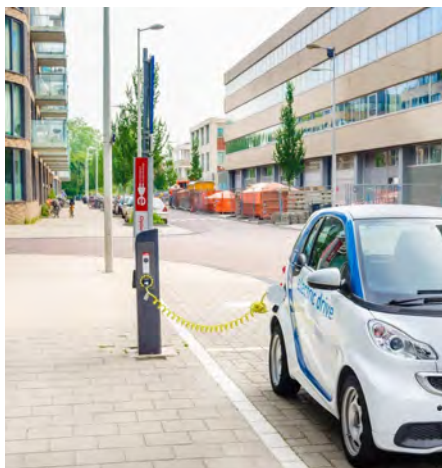
Electric vehicle charging points
